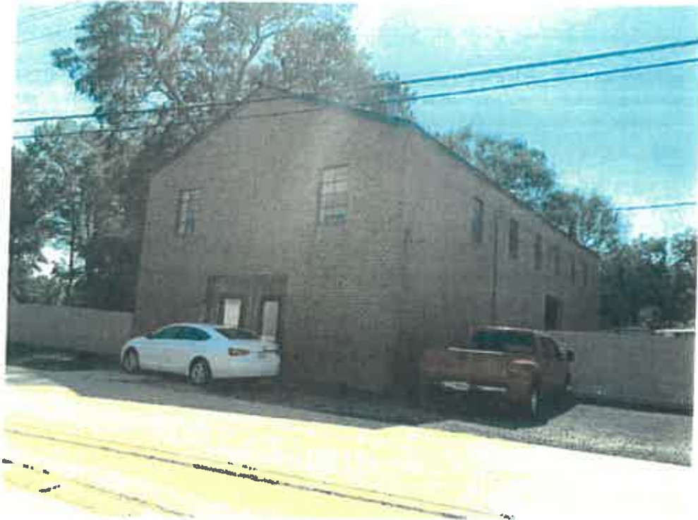
East and north facades
