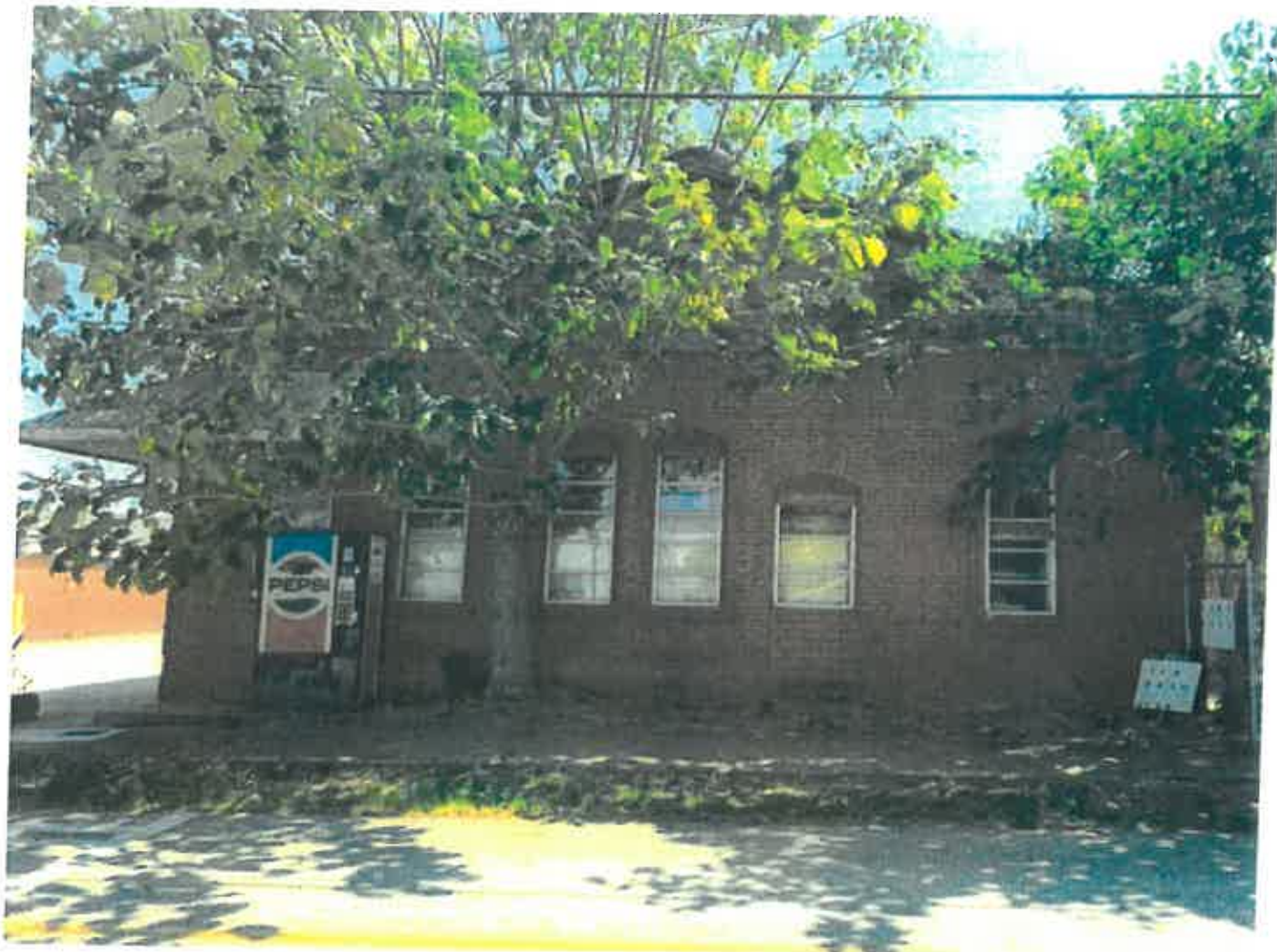
North Façade with wood shingles on gable.
