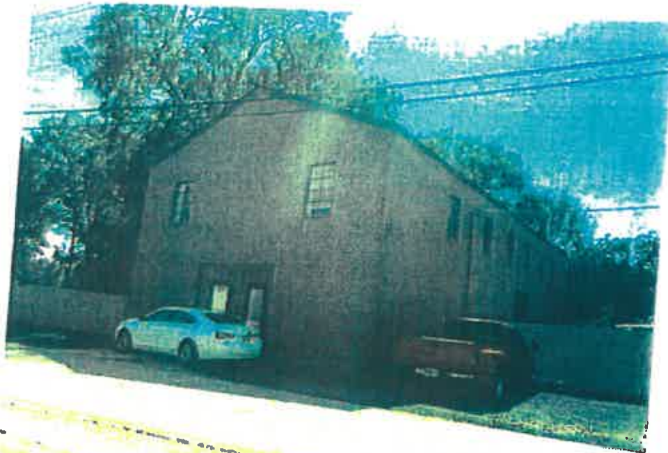
East and north facades
