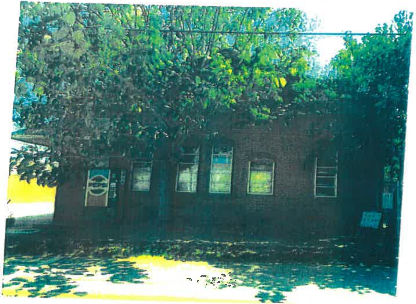
North Façade with wood shingles on gable.
