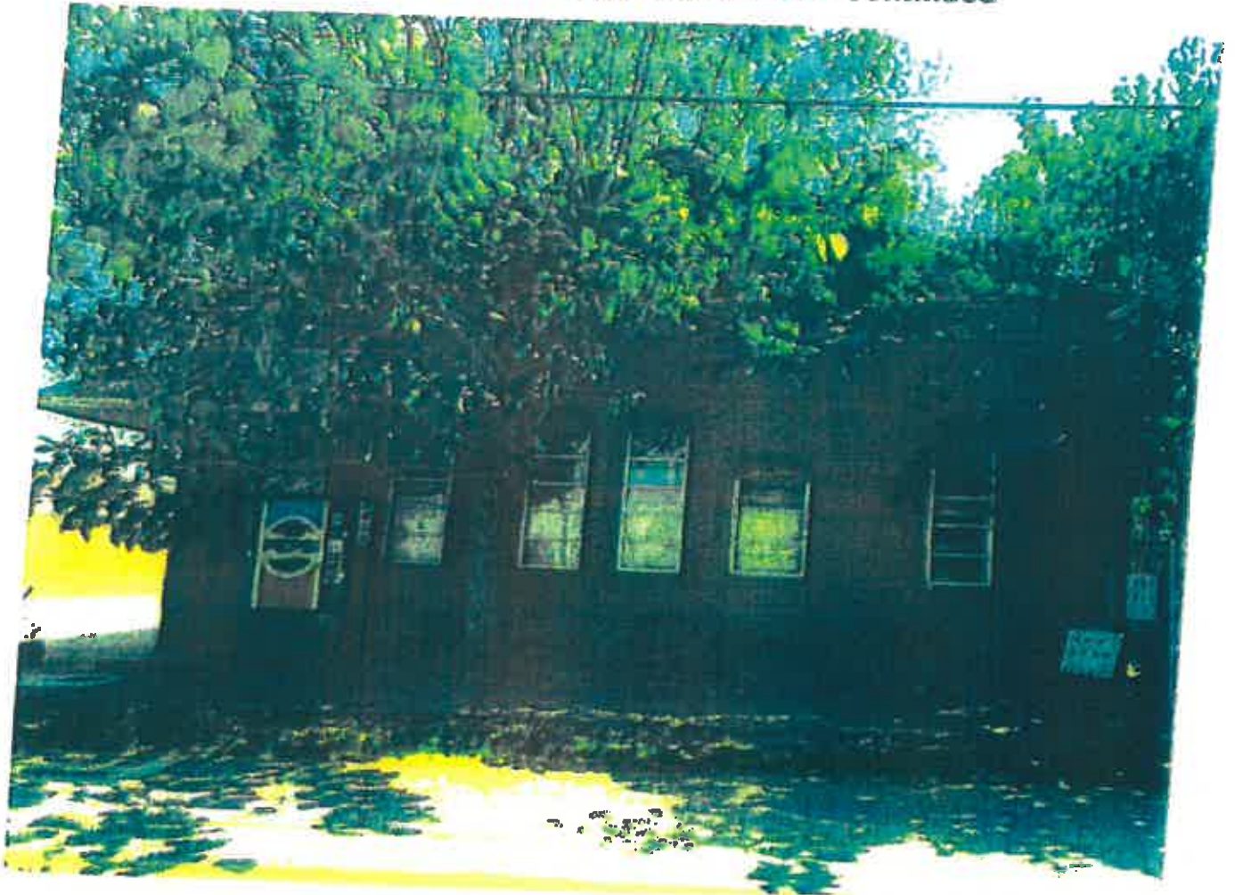
North Façade with wood shingles on gable.
