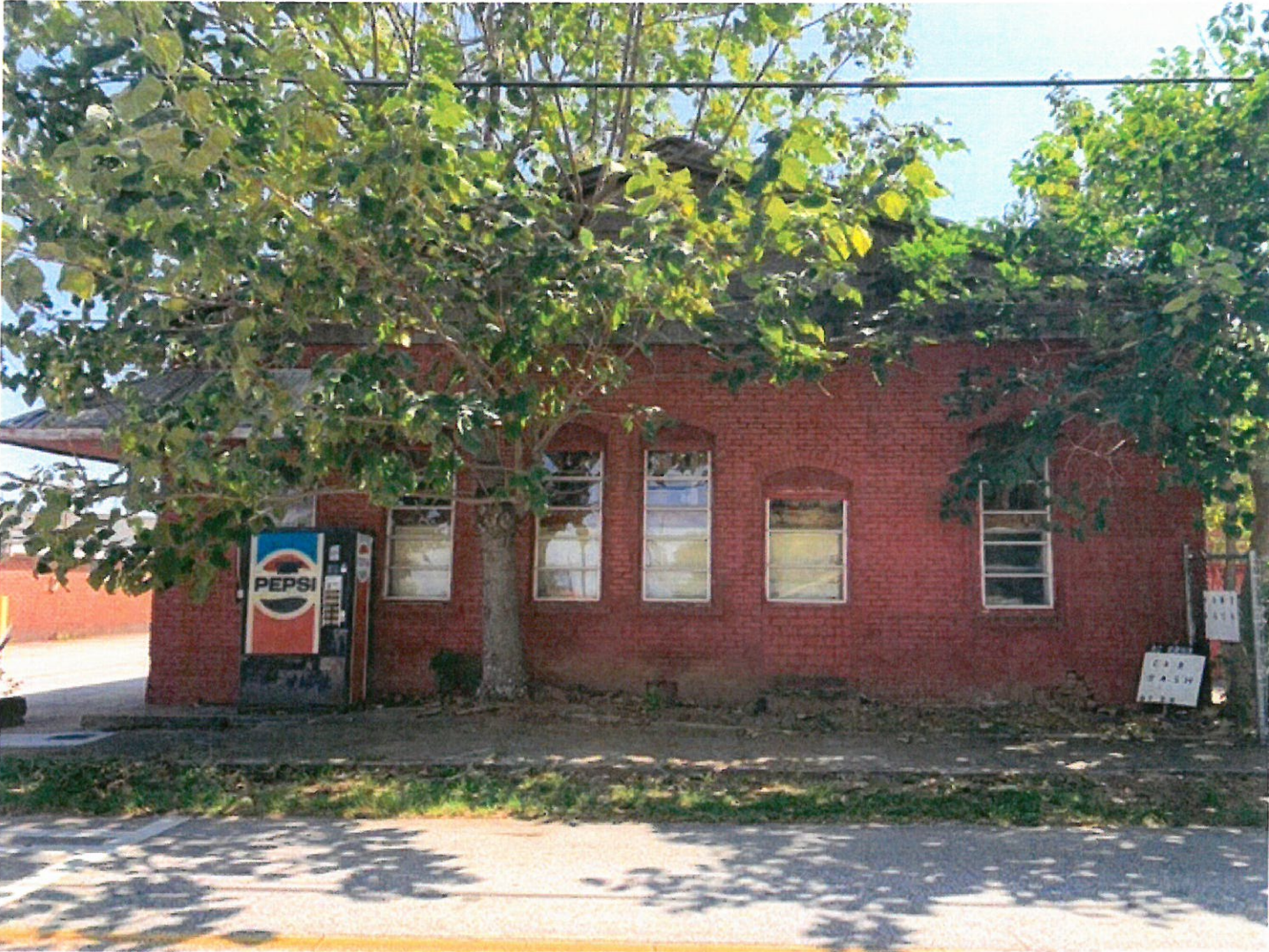
North Façade with wood shingles on gable.
