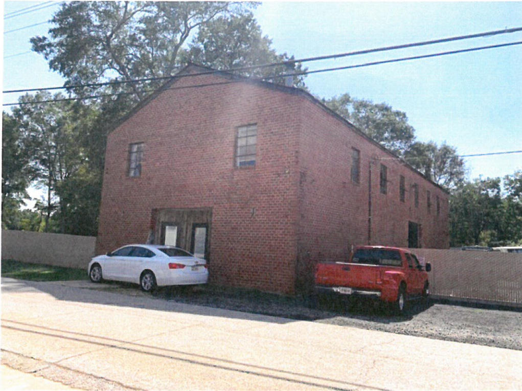
East and north facades
